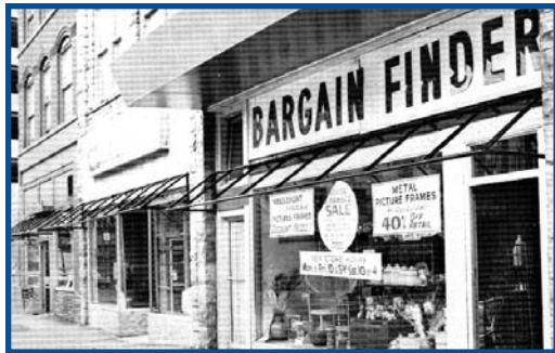
The 500 Block of Linden Street during renovation.
